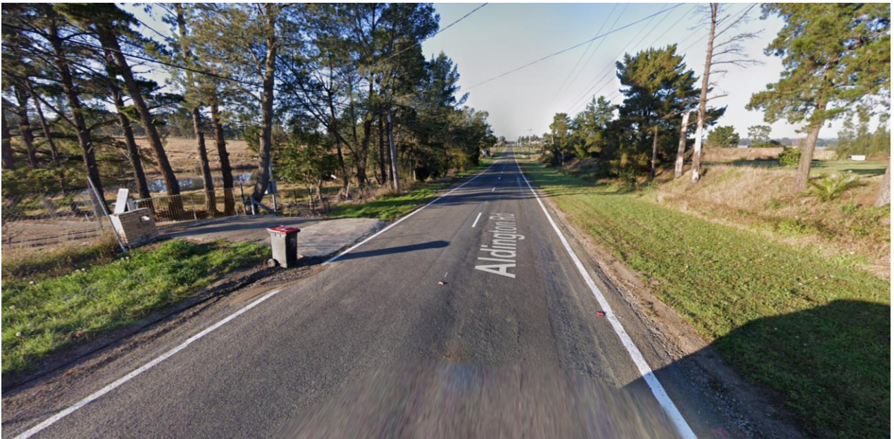
Figure 6: Existing northern Site Access, 244-256 Aldington Road (Source: Google Earth)
